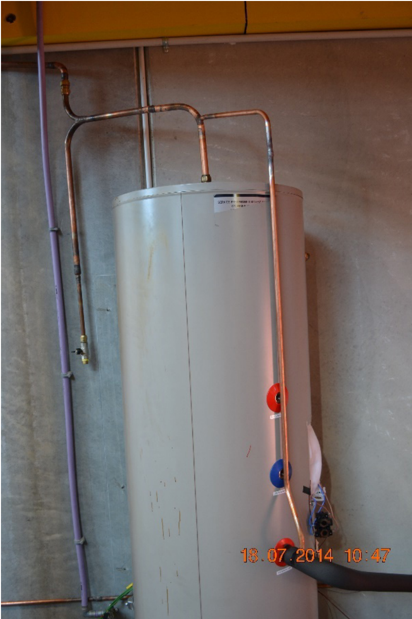
Figure 26. Stainless-steel indirect HWC, two coils.
