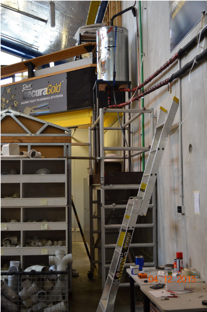
Water cylinder at 10 m distance raised 2.4 m above floor level.
